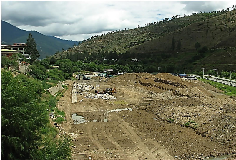
Formation cutting for the construction of Royal Craft Village and realignment of the expressway
